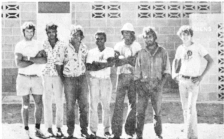
The men working on the site of the new caravan park to be set up at Wilcannia. On the extreme left is Billy Bates who will manage the park when it is completed. The other men in the photo, from left to right, are Charlis Dutton, Len Kerwin, Jim Wyman, John Wilson, Neville Bright, and Wayne Kirby
